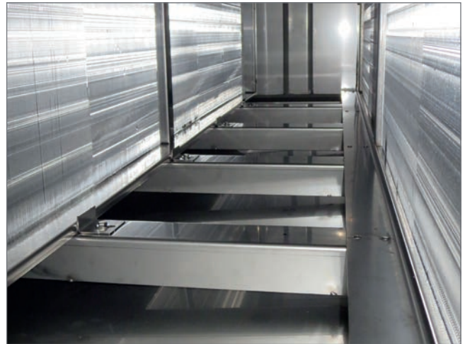
STAINLESS STEEL STRUCTURAL WORK
